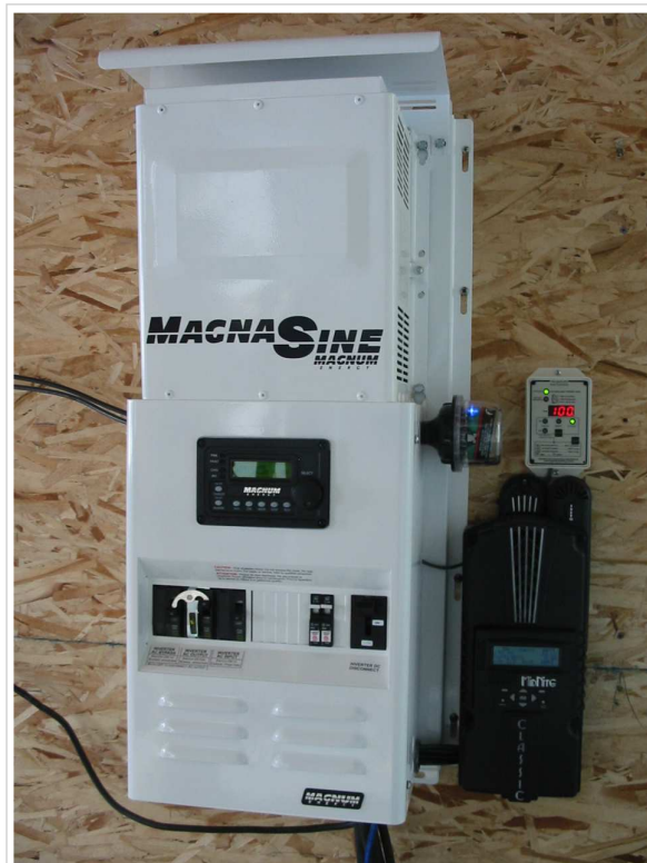
This is a power system. 4000 watts, 120/240V. That 100% is for 1200 amp hours at 24V.
