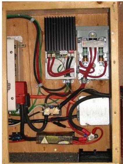
Tristar PWM, air conditioner disconnect, shunt for the Trimetric in the middle, inverter fuse at the bottom & inverter to left, insulated positive lug in lower right corner. AC power comes into the back of the 4x4 box on the right. It looks like spaghetti but this is just about the cleanest installation you will ever see and you can trace the wires. The batteries are through the wall on the right. (There Jim; now your rig is famous.) Warning: Do not buy the cheap air conditioner disconnect like this one if you are hooking up more than 25 amps. Find a Midwest Industries one. They are built a lot heavier.
