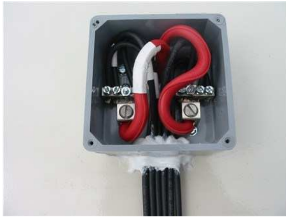
A simple cheap combiner box. All of the parts came from a big box store, and #4 booster cables from Walmart.
